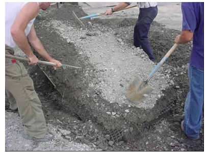
Compact aggregate using project-specific compaction equipment
