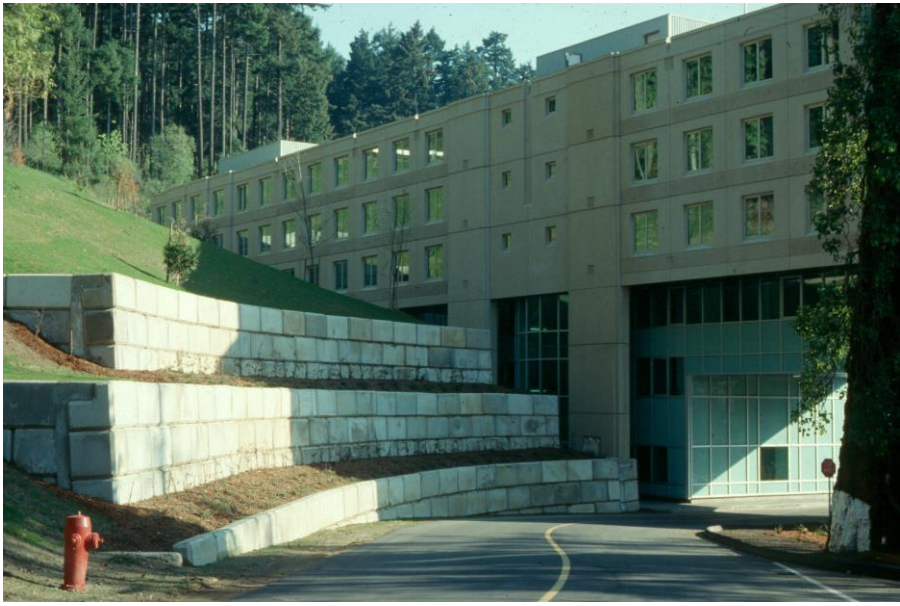
Royal Roads modular block wall (Victoria, BC, Canada)
