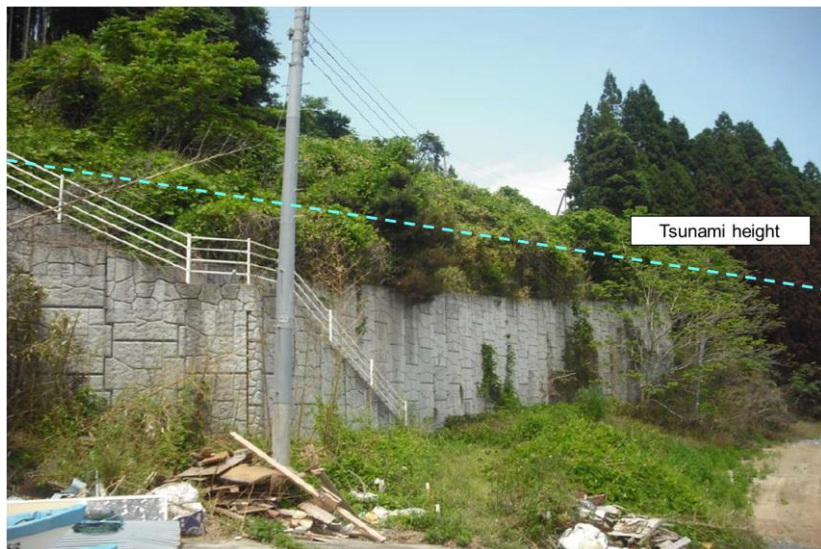
Photograph of 10.2m-high steel strip reinforced soil wall that survived transient flooding to depth of 14.9 m during 2011 tsunami (Rikuzentakata City, Japan).
