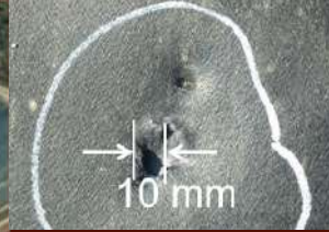
Longer-term stress crack
