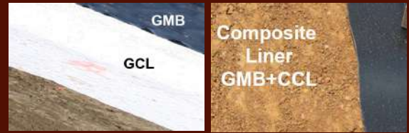
Barrier system with a single composite liner
